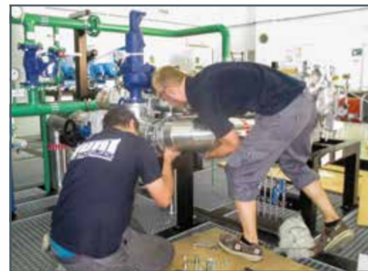
Assembly of the centrifugal pump on site
