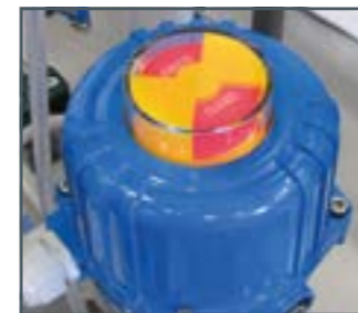
Electrically-driven ball valve
