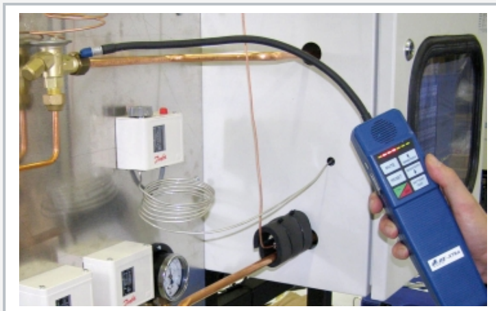
Leak test at the expansion valve of the fully assembled system
