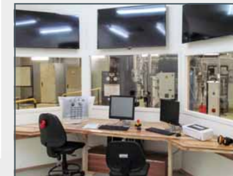
Module D control station
